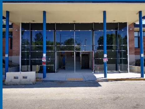
Continue Install of Curtainwall System and Glass at Entry
