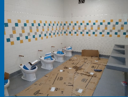
Install Toilet fixtures at Building 2010
