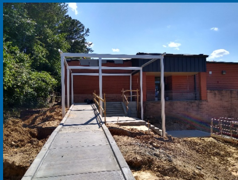
Begin Install of Canopy at ADA Ramp
